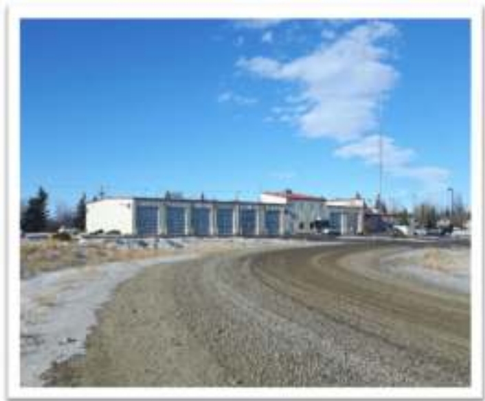
Looking northwest at the tri-services building
